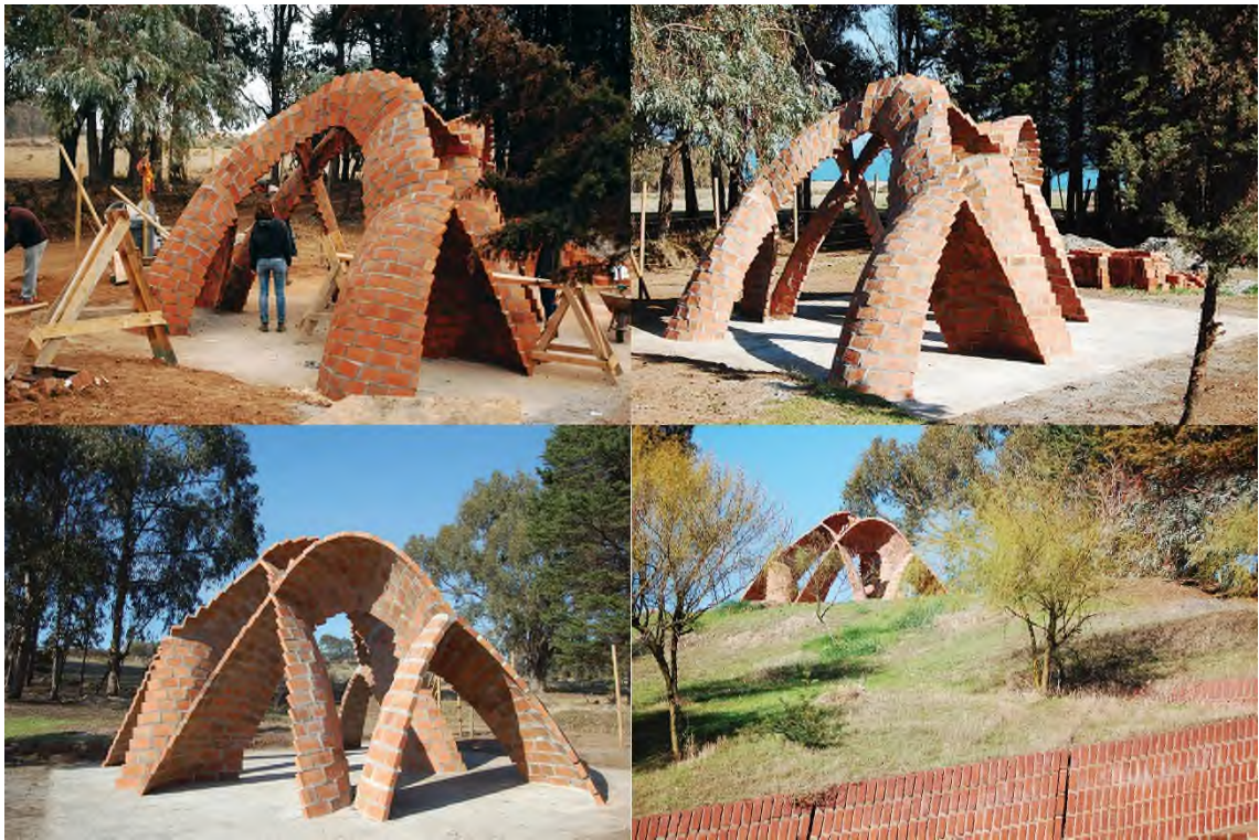
Figure 7 Nested Catenaries Workshop at e [ad] Escuela de Arquitectura y Diseño – Pontificia Universidad Católica de Valparaíso, conducted by Defne Sunguroğlu Hensel, engineer Guillem Baraut Bover and master mason Øyvind Buset, Open City, Ritoque, Chile, 2012 [Phase 3]: A Nested Catenaries Shell. This project was built as an extension to the cemetery of the Open City. The design constitutes 12 sub-shells of varying size, creating a volume of 162m 3 , each with synclastic surface curvature to retain the complexity of construction according to the allocated time.
